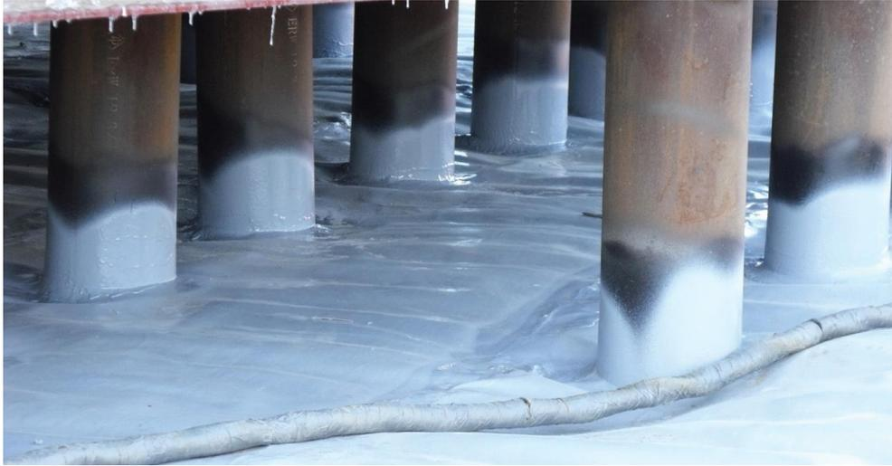
**Polyurea has excellent chemical and temperature resistance properties. As a Spray applied geomembrane polyurea can be modified for hardness, flexibility, chemical or UV resistance making it one of the most diverse geomembrane options available.**
