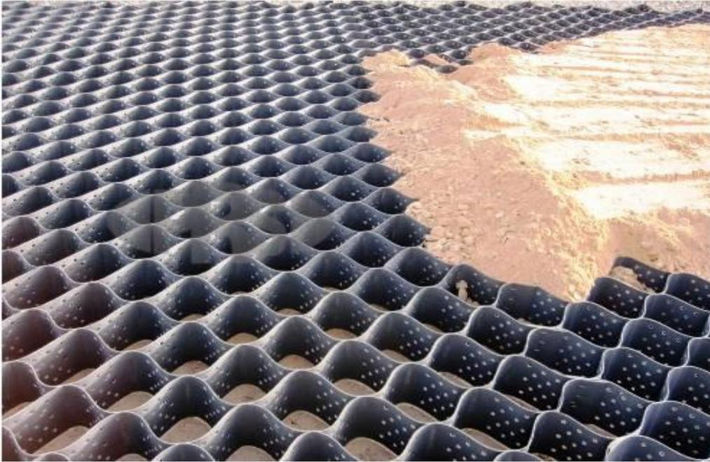
A variety of products exist which help prevent the erosion of soil through wind, rain or wave action. Depending on the application the solution may be as simple as an erosion control blanket or as robust as a cellular confinement product.
