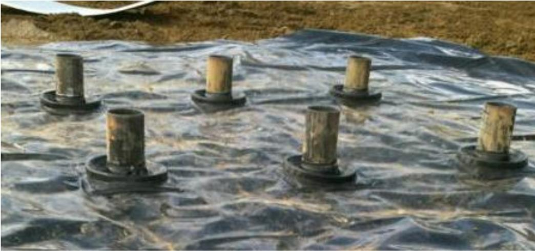
A common design feature of any secondary containment system is the use of posts or pilings to support the tank that will be providing the primary containment. However when this construction technique is utilized, an issue is how to best attach the geomembrane liner to any pilings that now penetrate the geomembrane liner.
