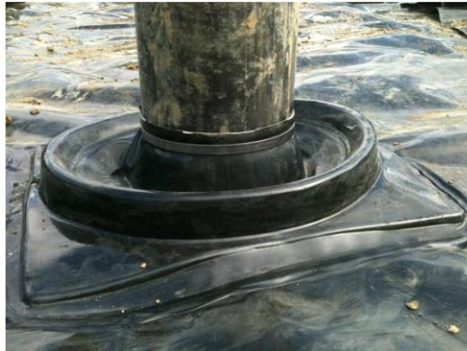
If settlement has occurred and the corrugations have been pulled up, we suggest that have our trained crews correct this deficiency. While the geomembrane in this area is still at its required thickness, this should not be viewed as a permanent solution to the issue.
