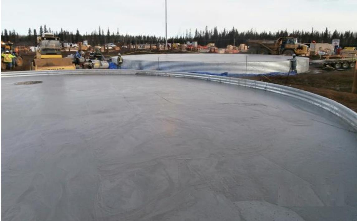
**The use of corrugated steel panels is an effective and cost-saving technique for the construction of gravel filled or concrete filled foundation rings**
