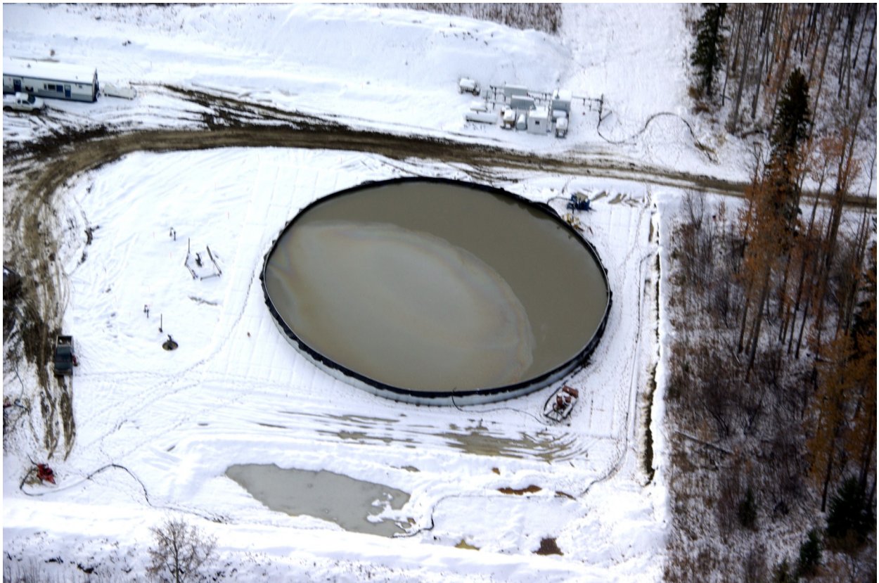
Frac Water Tank 138' Diameter x 7' 4" High Capacity: 3,076 m 3 Fort St. John, B.C.
