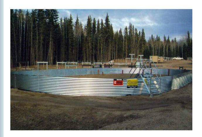
Secondary Containment System to Contain Two (2) 1,000 Bbl Tanks 41.8' x 55.8' x 44" High **Bottom Mount 40 mil LLDPE Liner Eight Liner Penetrations Crossover Stair**
