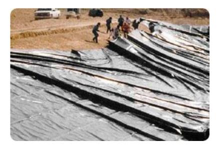
Woven Coated Polyethylene (WCPE) is constructed of woven, oriented tapes of HDPE. The tapes are then coated with a film of LLDPE which makes the liner impermeable to water and also gives the liner enhanced chemical resistance to hydrocarbons and other chemicals.
