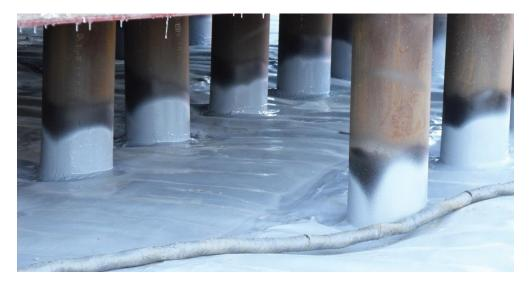
Polyurea has excellent chemical and temperature resistance properties. As a Spray applied geomembrane polyurea can be modified for hardness, flexibility, chemical or UV resistance making it one of the most diverse geomembrane options available.
